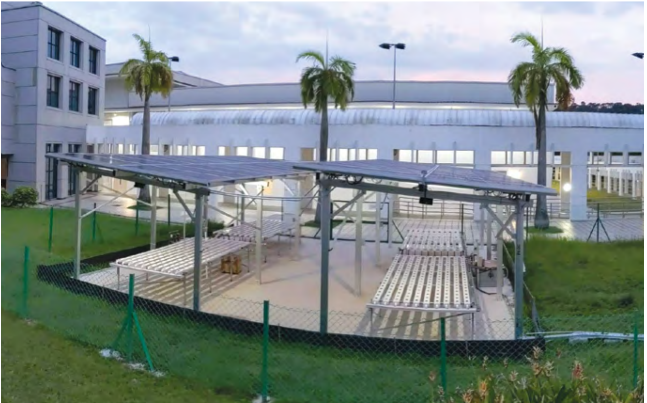
An agrivoltaic system, with the solar PV panels installed on the roofs of the sheds, and the setup for the growth of hydroponic plants installed within the sheds.
