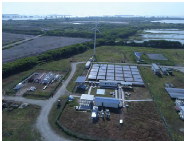
ENGIE's testing facilities on Pulau Semakau features Singapore's tallest wind turbine, a solar farm, a battery storage system, and a green hydrogen full value chain.
